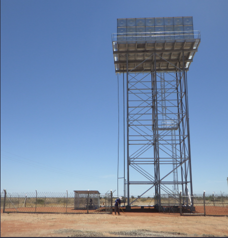
Stampriet Service Phase 4 - Water Tower
