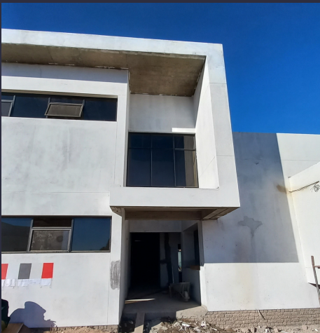
Oranjemund Fire Station
